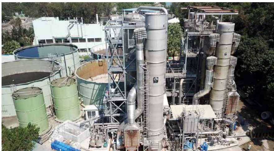
The 3,250 m 3 /day rated thermal ammonia stripping plant at the West New Territories (WENT) landfill site, Hong Kong, China.
